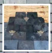
Snow guards are installed in rows in a staggered pattern along the eaves of a roof.
